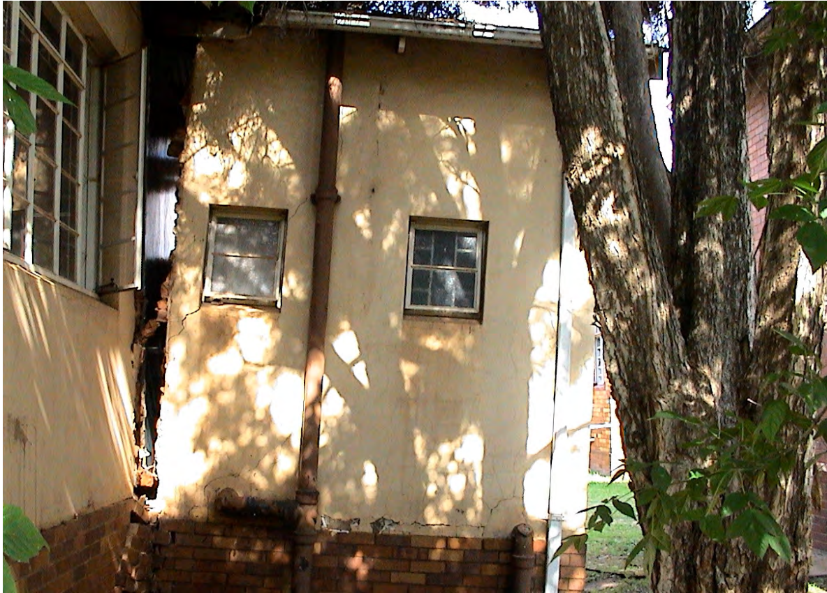
PLATE 8: BUILDING MOVEMENT AS RESULT OF DOLINE
