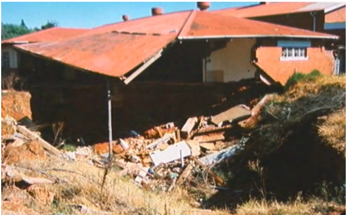
PLATE 6: SINKHOLE AS RESULT OF LEAKING WET SERVICE
