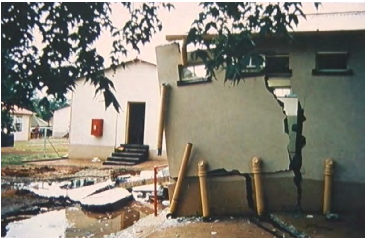
PLATE 9: BUILDING MOVEMENT AS RESULT OF DOLINE FORMATION
