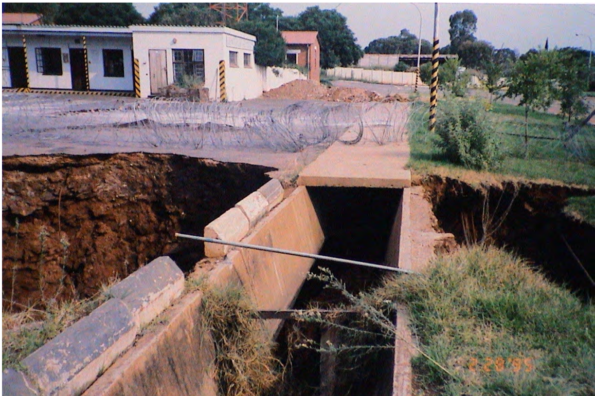
PLATE 2: SINKHOLE AS RESULT OF LEAKING STORM WATER CANAL
